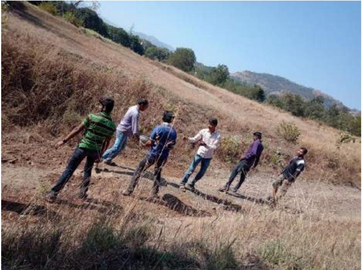
Construction of road at Andgaonvillage DEC 2017
