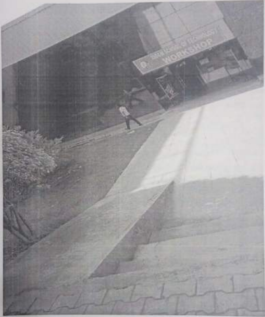
RAMP FOR TOWARDS WORKSHOP
